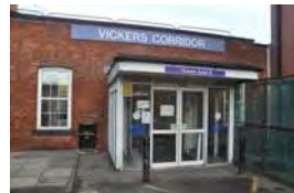
20 Access to Vickers Corridor and wards
